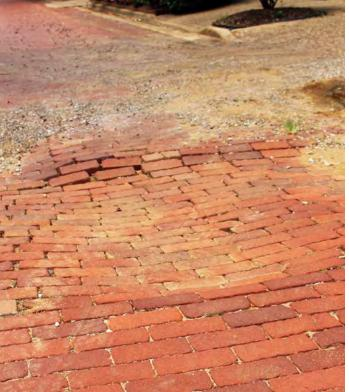
'Pothole of the Week' is back. The Gladeater Mirror's weekly feature focuses on streets in serious need of repair. This week's featured problem is an oldie, but a goodie on Quitman Street. A waterline rests under these sunken bricks and every time large trucks pound these bricks, the waterline has to be taking a beating. No asphalt is needed to fix this - just some dirt and time.
